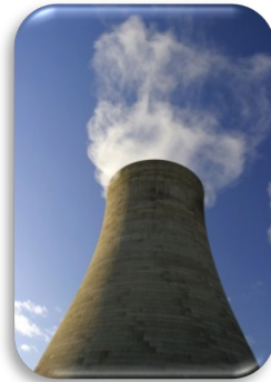
Nuclear Power Plant
