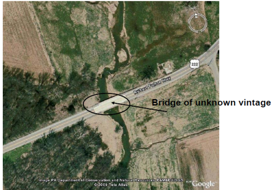
Figure 6-16 Bridge along Robert Fulton Highway
